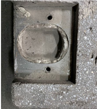
Before hinge installation
